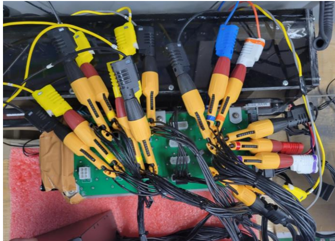
Figure 3: Insulated Piercing Probe to Measure the Output Voltage of Desktop Power Supply
