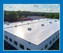
Like insulation, a cool roof reduces the amount of cooling needed by decreasing the heat transferred into the building and surrounding environment. Flat roof insulation prevents air leaks – a leading cause of energy waste in most commercial buildings.
