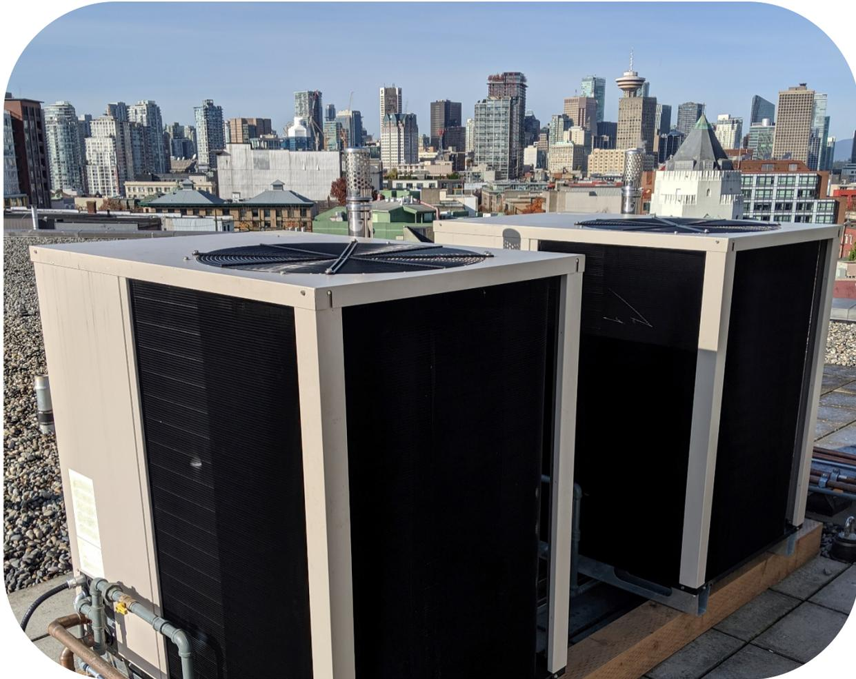
*Image: GAHP units being commissioned at a facility for a FortisBC pilot project in Vancouver, British Columbia. Courtesy of Building Energy Solutions Ltd.*
