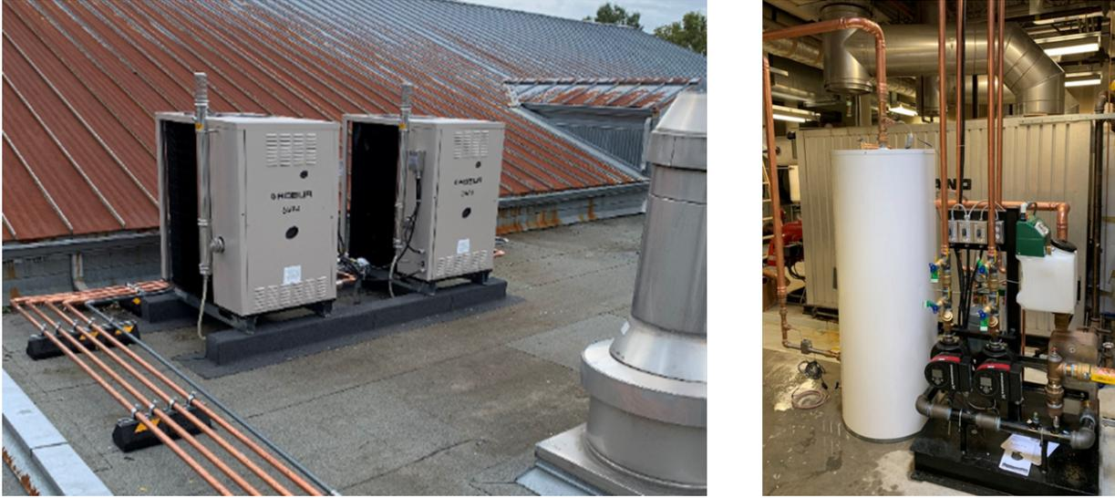
**Figure 3: Left: Robur GAHP-A units installed on a rooftop. Right: Pump skid with a buffer tank and glycol feeder**
